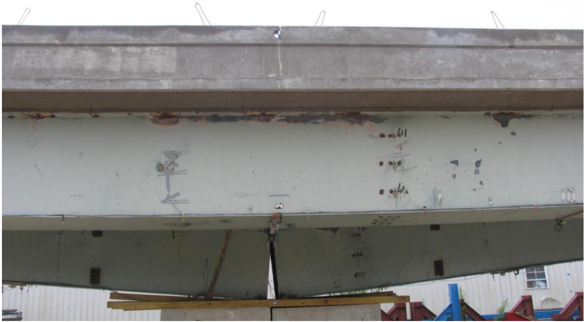
Figure 15. Side view of intact girder.
