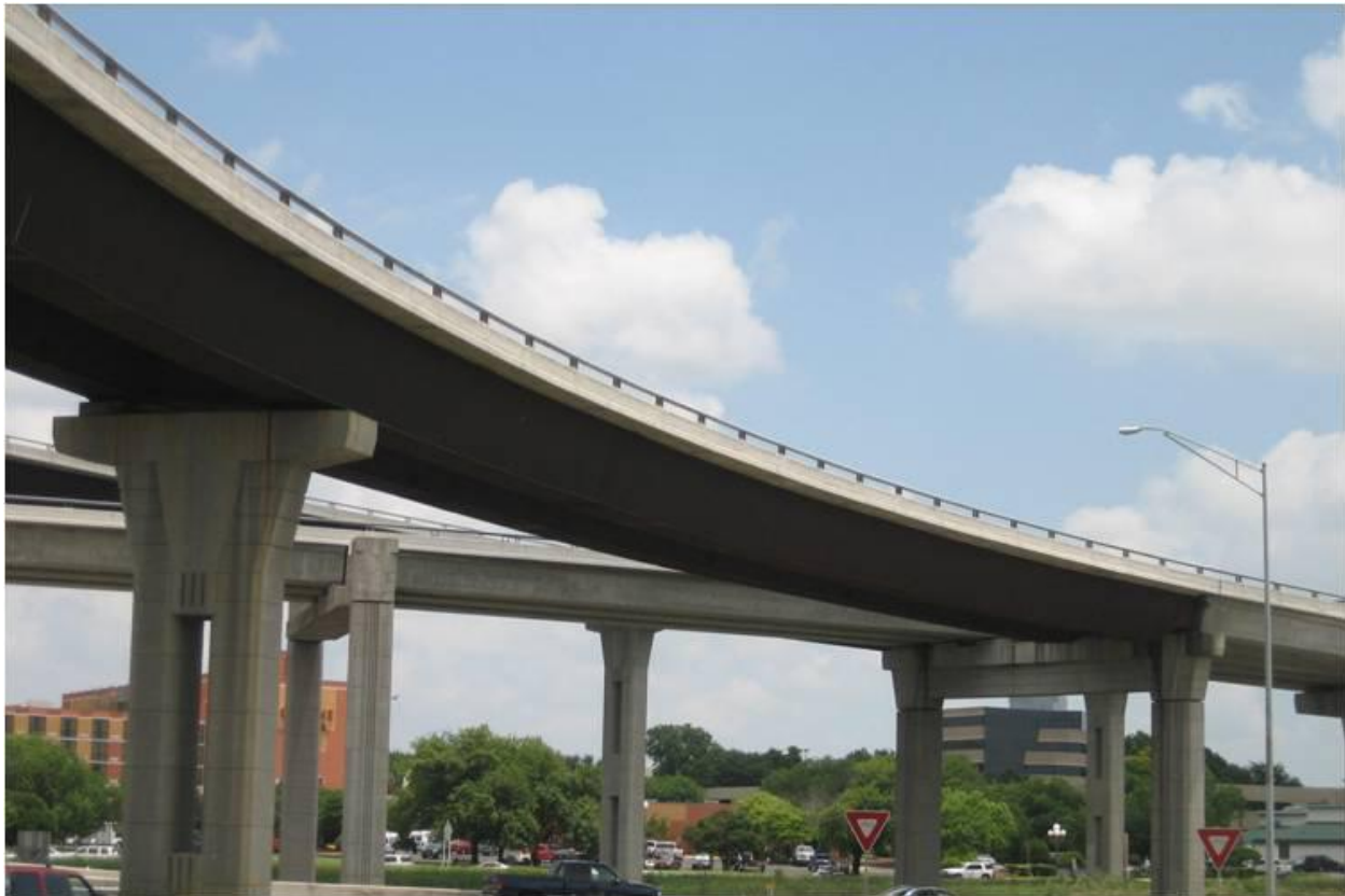
Figure 1. Twin box-girder steel bridge (Ferguson Structural Engineering Laboratory)
