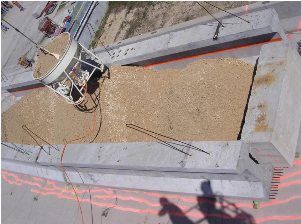
Figure 11. Loading the bridge with road base.
